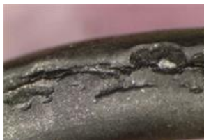
Thermal degradation of elastomeric seals
